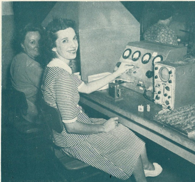
TESTING SELENIUM RECTIFIERS. Helen LeMay (right) testing and Helen Dealy painting. The selenium rectifier can be seen at the right. — BOSTON ELECTRONICS.
