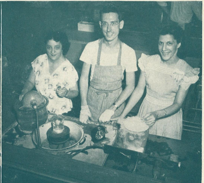
TR BOXES tested in hot and cold water. Cold water at right is kept near freezing point with dry ice. Left to right, Rose Cangiano, John Higgins and Nellie Goodman. — BOSTON ELECTRONICS.
